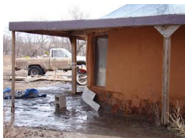
Pic. 8. A low base and a slope from the house can be disastrous when spring flood or abnormal rainfall.
