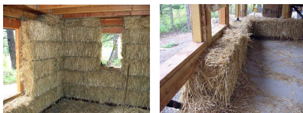
Pic. 23-24. Arrangement of walls and window openings
