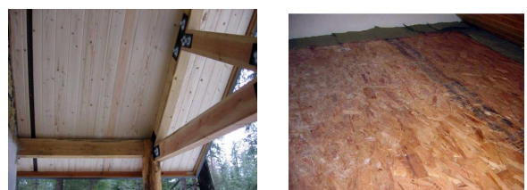
Pic. 28. Ceilings and a roof in the house of straw are sheathed with lining
