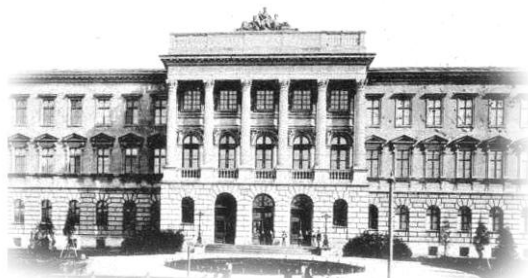
The main building of Lviv Polytechnic
