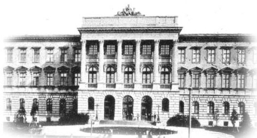
The main building of Lviv Polytechnic
