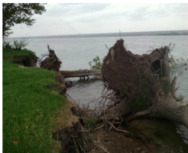
Fig. 8. Degradation of shores due to wave erosion and tree weight
