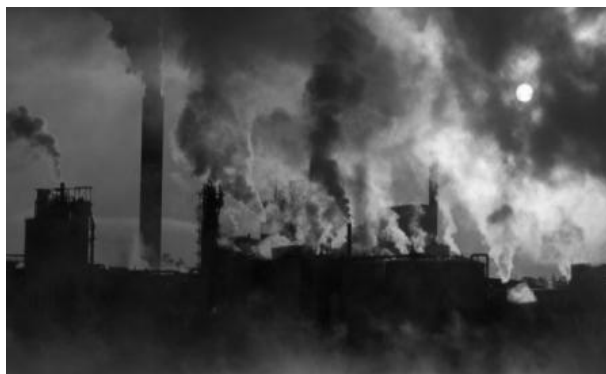
Fig. 1. “Panorama” of the metallurgical plant OJSC “Arcelor Mittal Kryviy Rih”
