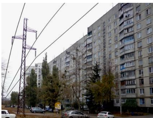
Fig. 1. The location of a 110 kV overhead power line with triangular phase conductors arrangements.
