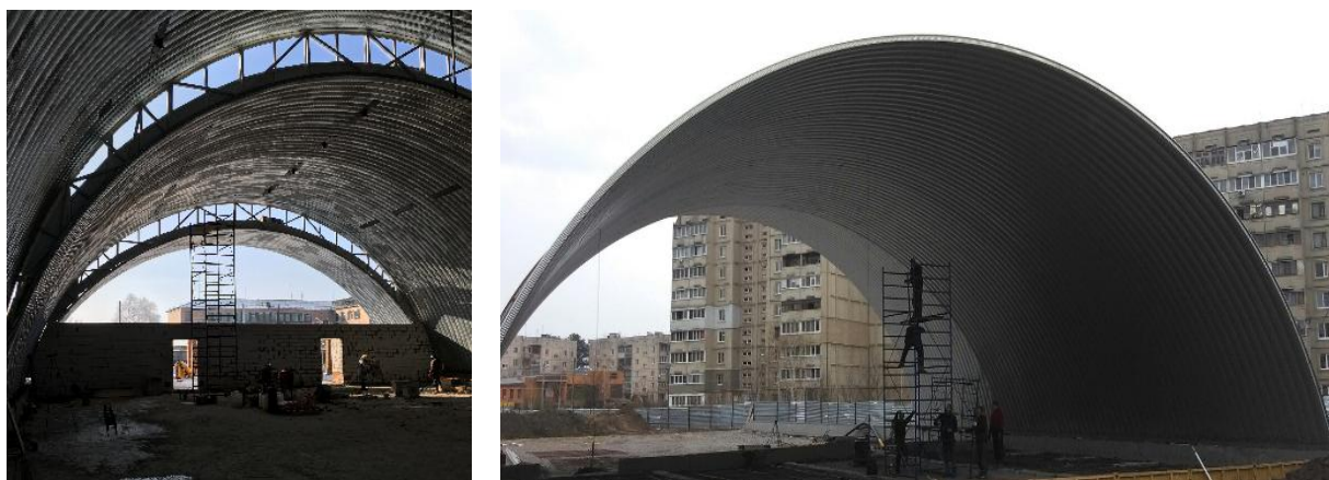
Fig. 1. An example of a special-type arch covering erection
