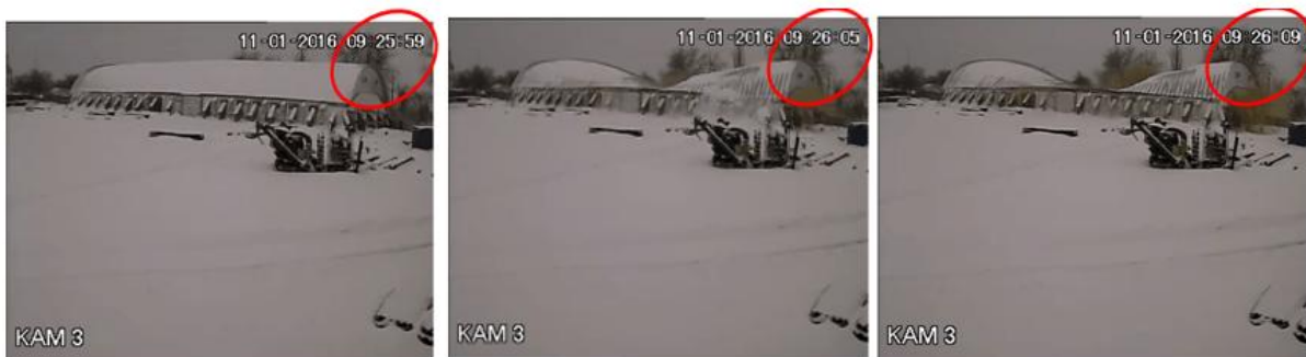
Fig. 2. Progressive collapse of a special-type arch structure
