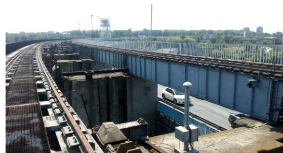
b – monitoring point MP-4
