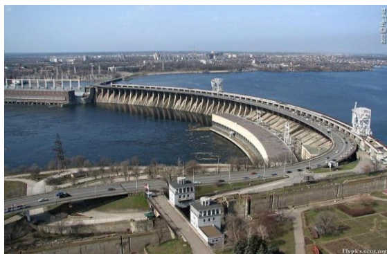
Fig. 2. Drainage dam of the Dnipro HPP.
