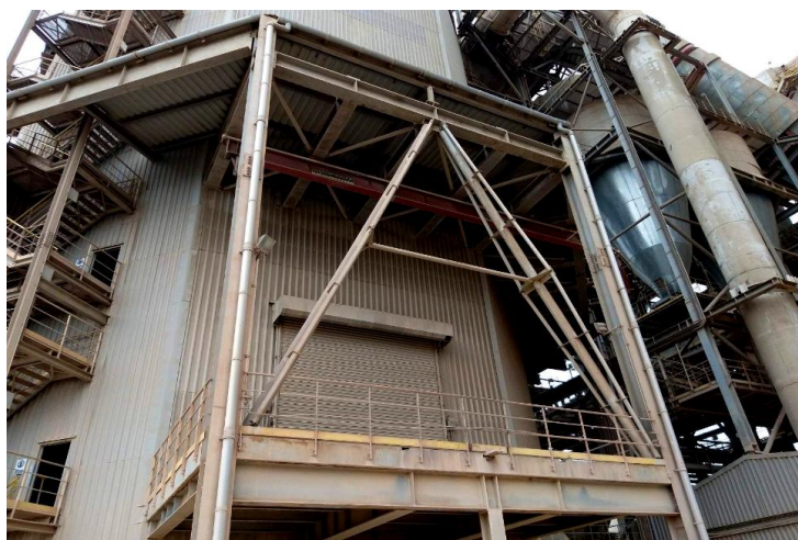
Fig. 6. General view of structures after reinforcement under load
