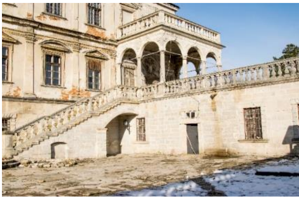
Fig.13. Photo of the terrace that is formed by casemates in Pidhirtsi bastion castle (Author's photo)
