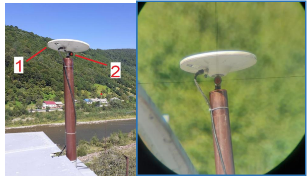
Fig. 8. Continuous GNSS station TERE 1 – GNSS antenna, 2 – reflector
