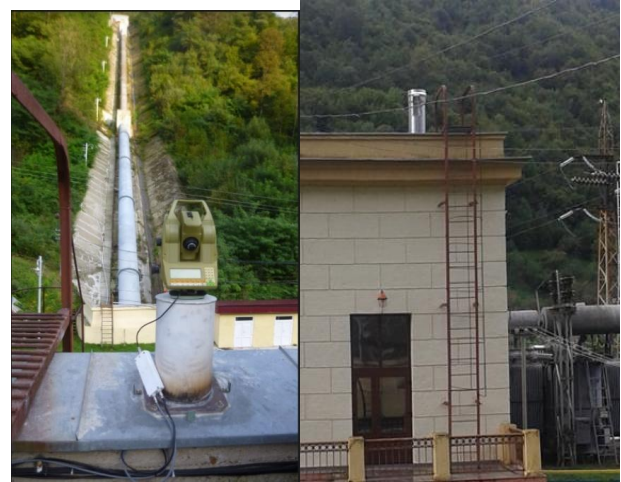
Fig. 4. Robotic total station LEICA TPS1000 with thermal protection installed on the roof of the generator hall
