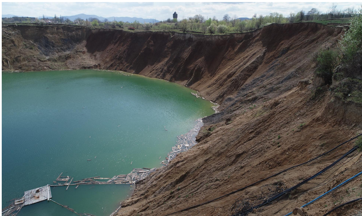
Fig. 1. Flooded mine No. 7
