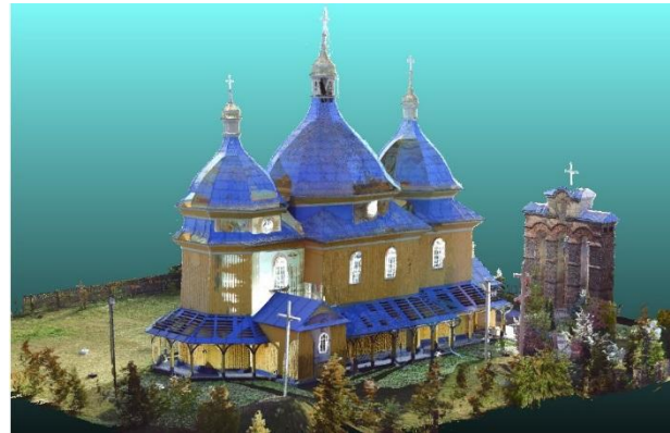
Fig. 3. Cloud points of the scanned church Sushno village Lviv region
