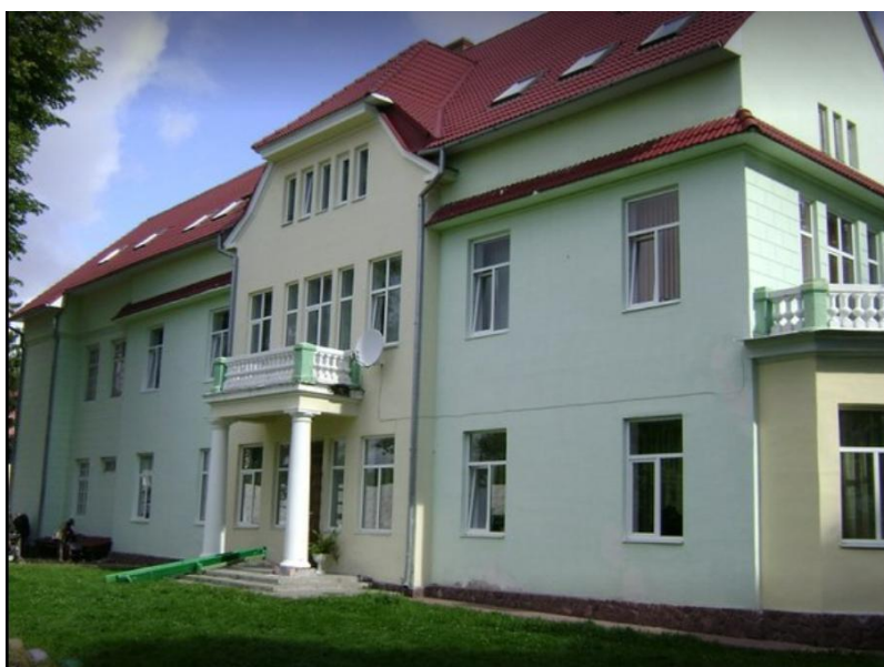
Fig. 1. General view of the school building. (Source: https://www.google.com/maps/ )
