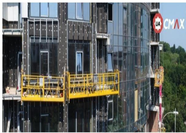
Fig. 2. Installation of glass blocks and elements for the realization of modern buildings
