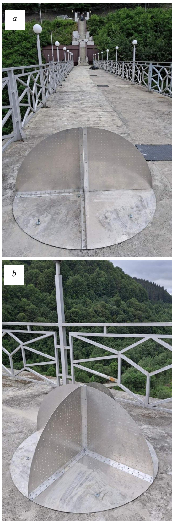
Fig. 7. The quadruple corner reflector with 1.0 m inner leg length, deployed at the dam of Tereble-Ritska HPP: a) view 1; b) view 2
