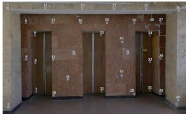
Fig. 1. The survey area located in the hall of the FGI department
