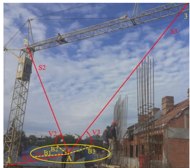
Fig. 3. Illustration of ET measurements of angles and lines to points on a tower crane
