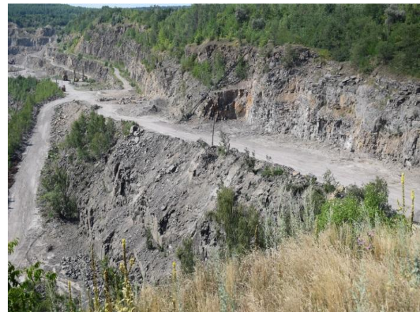
Fig. 7. Current active development of landslide processes in the northern part of the western wall of the Hnivanskyi quarry.
