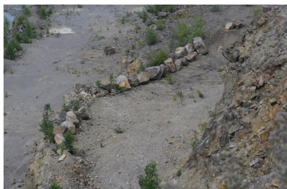
Fig. 6. Safety shaft on the quarry road (southern part of the Hnivanskyi quarry).
