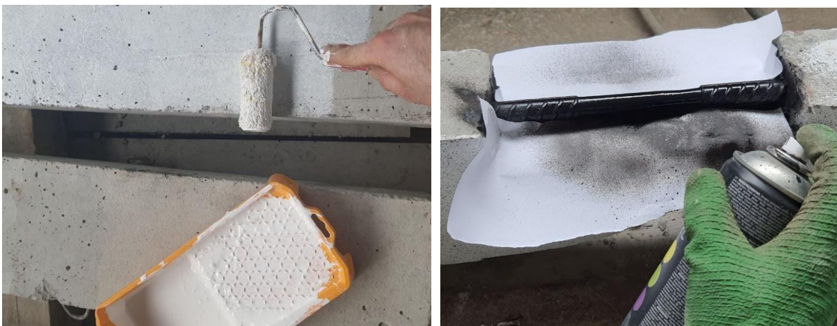
Fig. 2. Application of a white background on concrete (left) and a black background on reinforcement (right).
