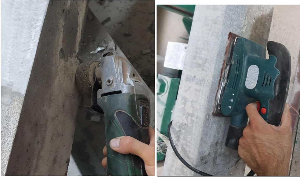
Fig. 1. The process of leveling and cleaning the surface of concrete and reinforcement.
