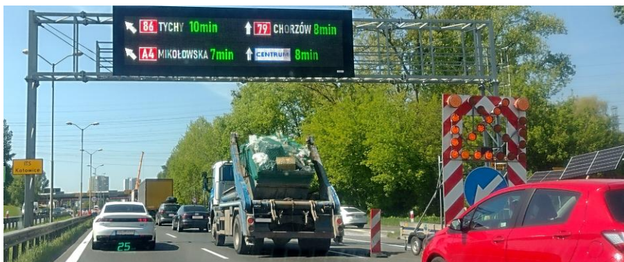
Fig. 2. Variable message board of the discussed “ITS Katowice” system displaying travel times to selected points of interest, i.e., the neighboring cities “TYCHY” and “CHORZÓW”, and to the intersection with MIKOŁOWSKA Street.
