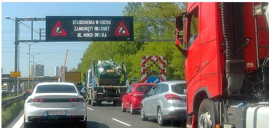
Fig. 1. Variable message board of the discussed “ITS Katowice” system with the displayed information “TRAFFIC DISRUPTIONS, CLOSED VIADUCT ON MIKOŁOWSKA Street”
