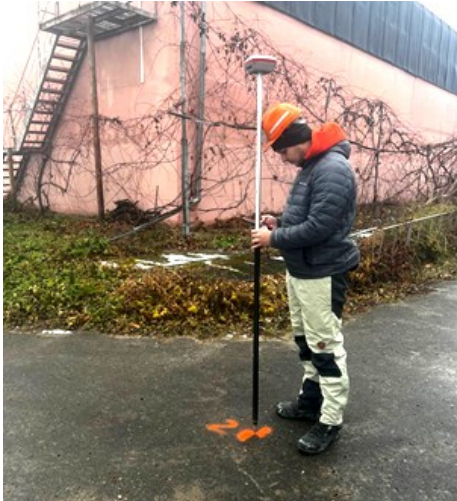
Fig. 3. Recording the coordinates of control points – item 2
