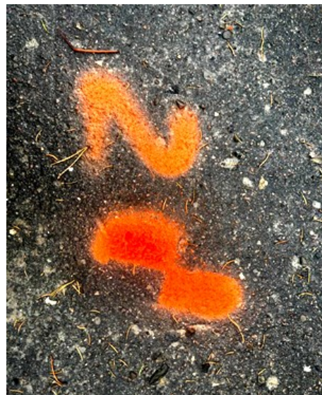
Fig. 1. Marking control points with paint
