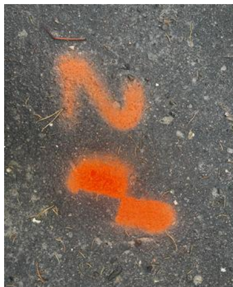
Fig. 1. Marking control points with paint
