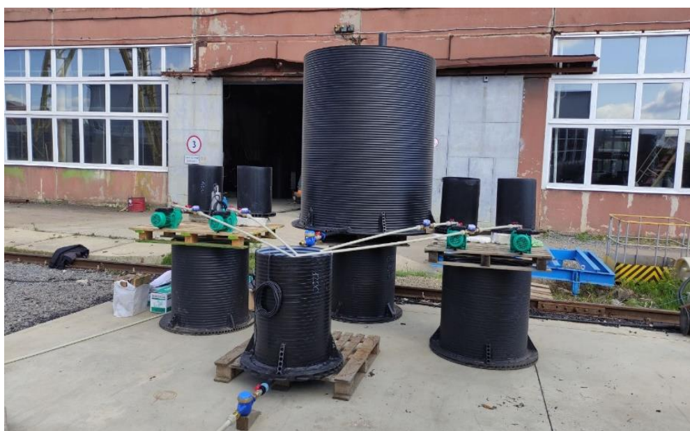
Fig. 2. Pilot leachate treatment plant at the pre-assembly stage (Energoresurs-Invest Corporation, Lviv)
